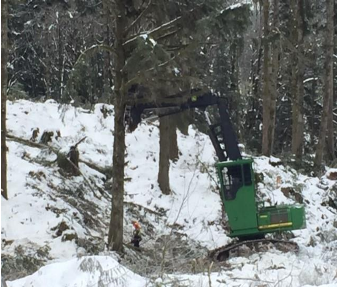
West Coast Operations – Block 173118 – Assisted Falling for Power Lines
